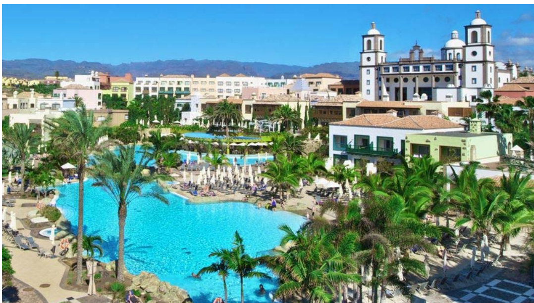
Session A: Located in the last floor of the main building
